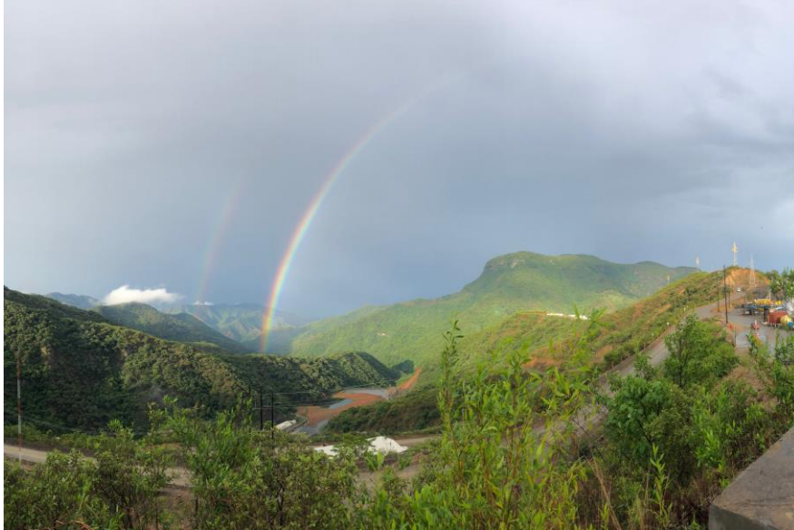
Campo Morado looking SE over Abajo tailings storage facility
